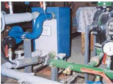
Fig. 1.3: Installation of an Acoustics-T device on a plate heat exchanger.
