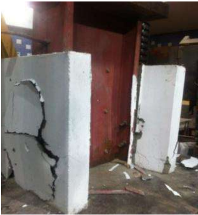
Fig. 6(b): Crack on slabs.
