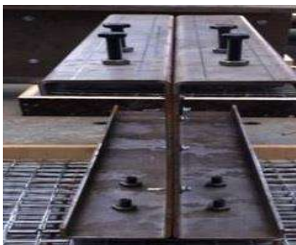
Fig. 2: Fixing shear connectors.
