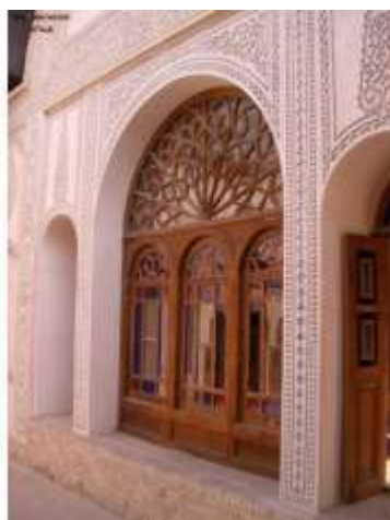
Figure (8): Tabataba'ees' House sash window, source: Isfahan cultural heritage office
