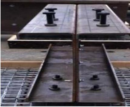
Fig. 2: Fixing shear connectors.
