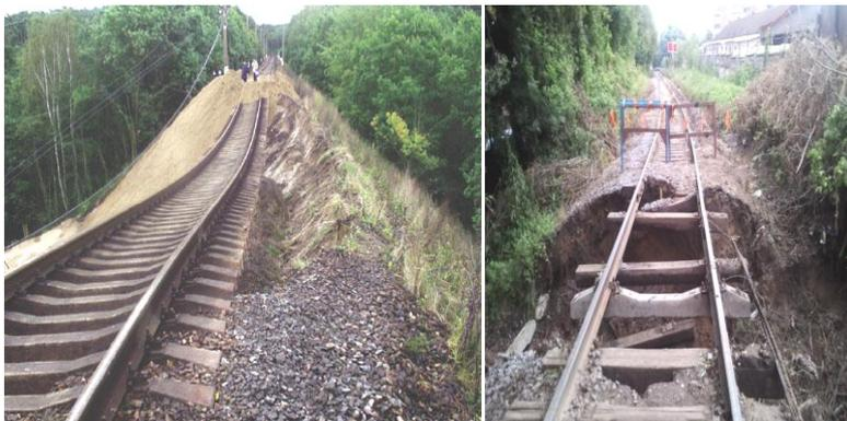
**Fig. 1:** The sudden destruction of the subgrade of the railway as a result of natural factors
